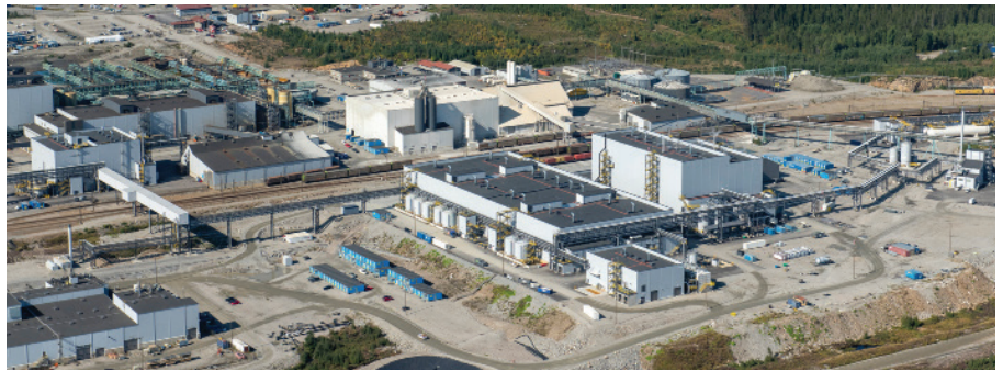
The battery chemical plant is located in the Terraframe factory area
