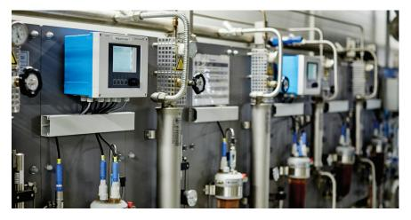
Endress+Hauser and Alfa Laval Aalborg have developed a steam and water analysis system (SWAS) that meets their clients' needs. The solution is currently showcased and in use at the Alfa Laval Training Center in Rauma, where Alfa Laval's Finnish and international clients can come and see it.
